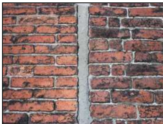
Brickwork of the lengthman's cottage (1779) and toll house (1795).
