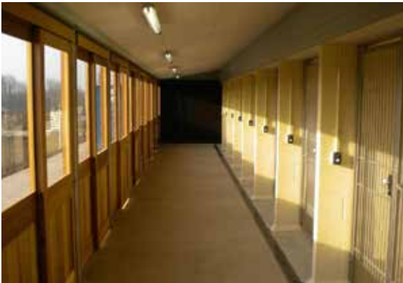
Kennel runs (corridor and screens)
