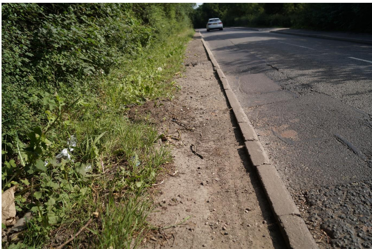
Photo 13 illustrates the damaged verge along Ilkeston Road caused by vehicles mounting it due to the narrowness of the carriageway
