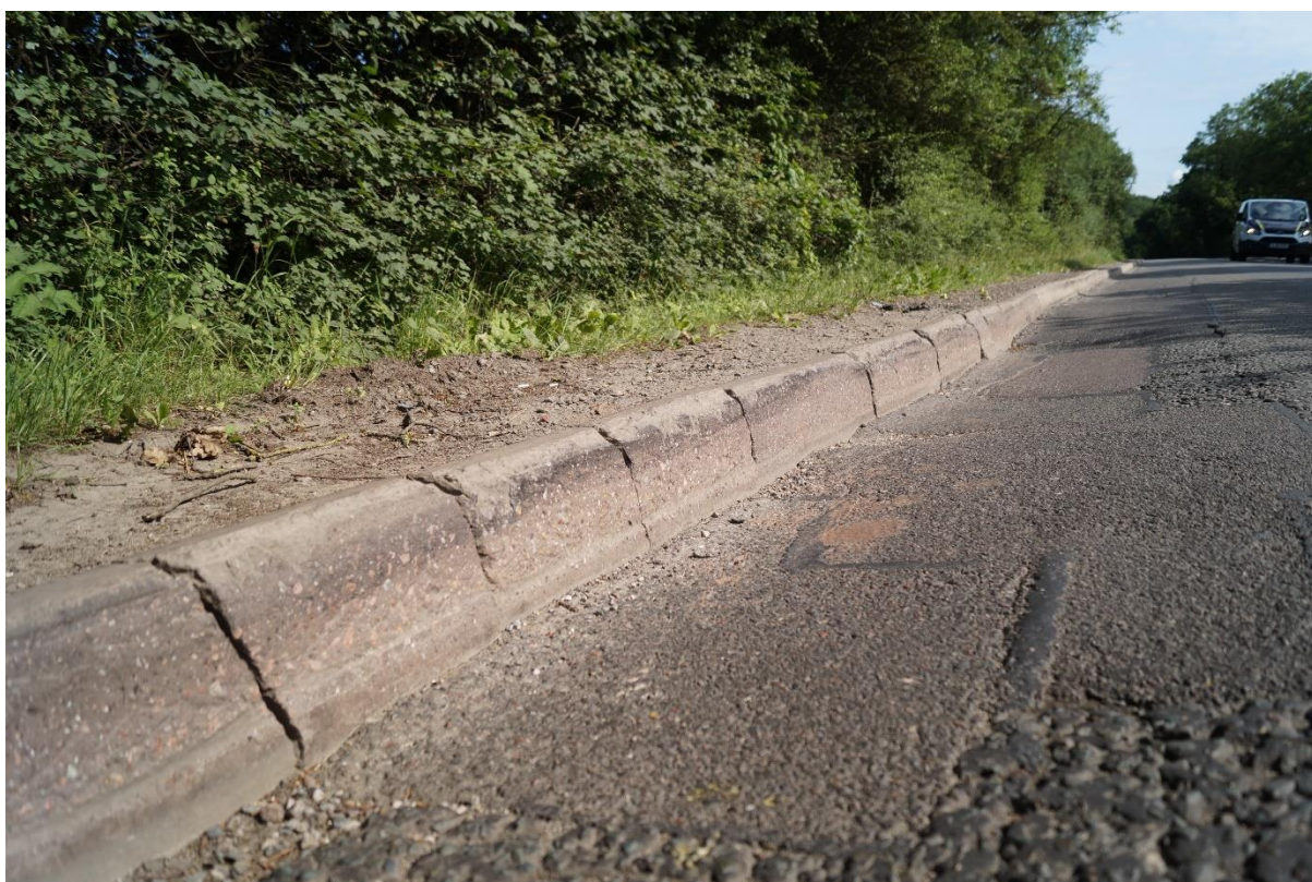
Photo 14 illustrates the damaged kerb along Ilkeston Road caused by vehicles mounting it due to the narrowness of the carriageway
