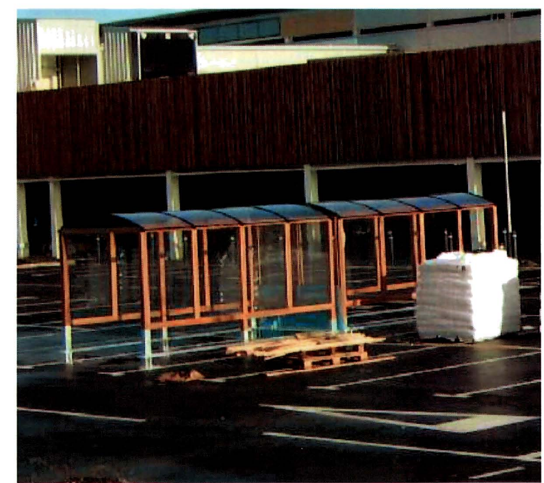
PHOTO SHOWING TYPICAL TROLLEY BAY
